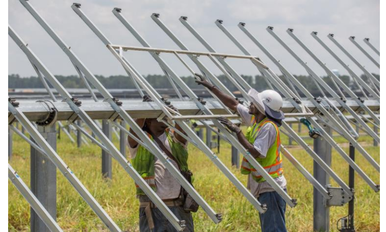
3) Installing racking
