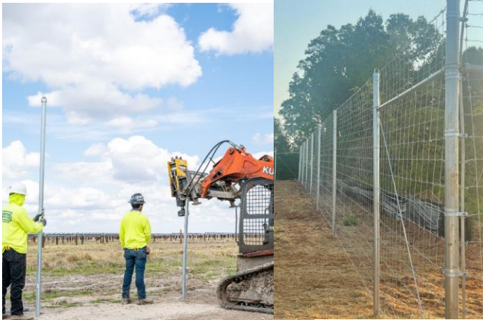
1) Installing perimeter fence
