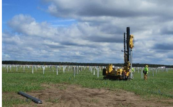
2) Drilling and pounding posts
